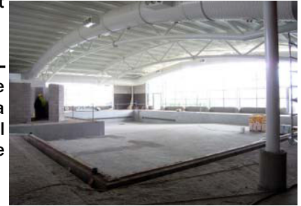
Progress with construction of North Herefordshire Swimming Pool
